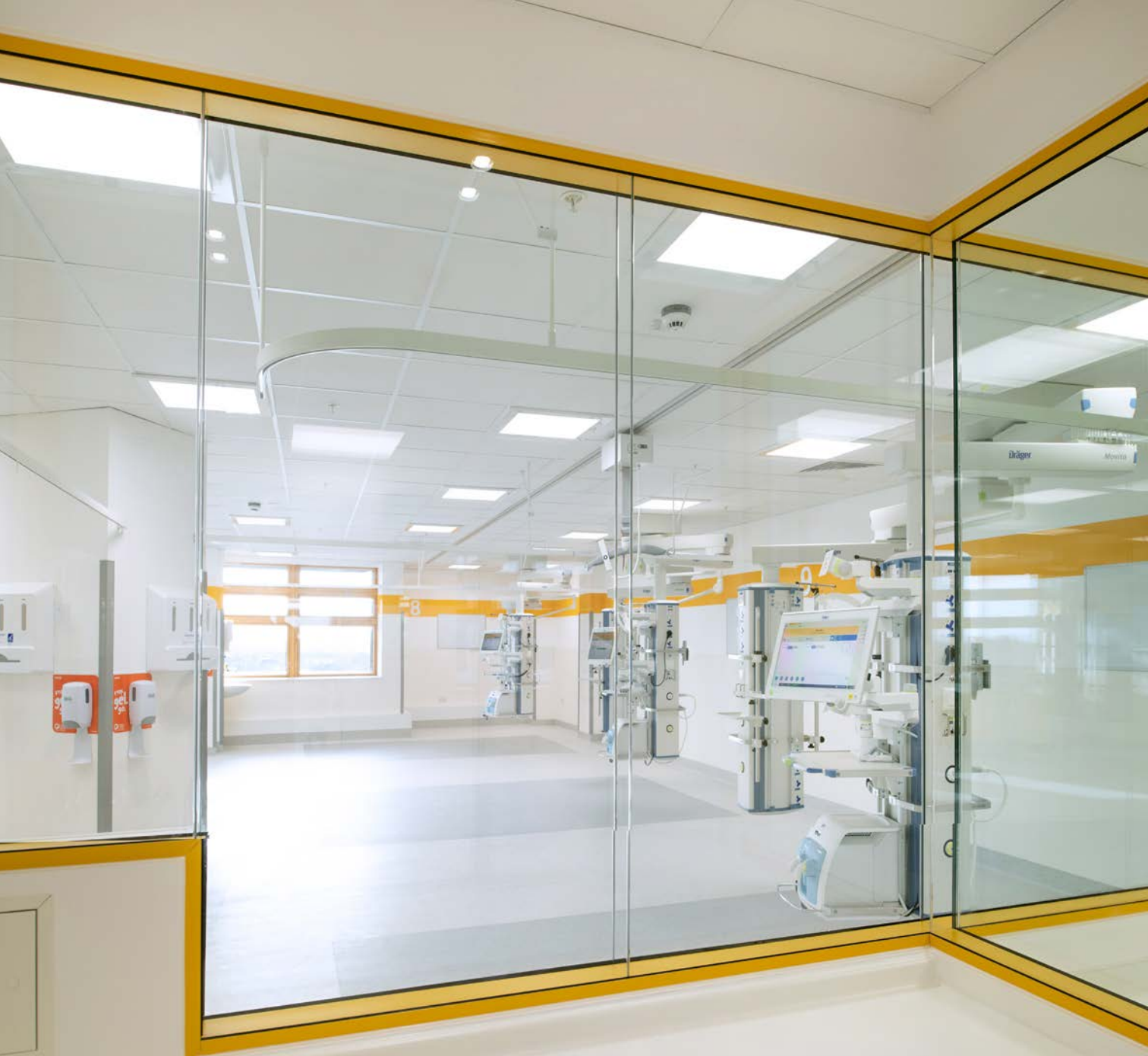
Barking, Havering and Redbridge University Hospitals: Queens Hospital Critical Care Unit
