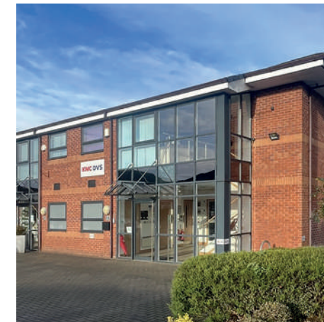
KWC DVS Northern Office, Chesterfield, UK
