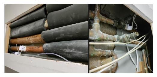
The recirculation pipework temperatures are below, first for the corridor outside room 11 and then also the pipework monitored in the second picture near room 1 (next page). The temperatures in the main pipework run appear to be reaching 55, however they are not staying above this level. The probe by room 1 shows temperatures well below this.
